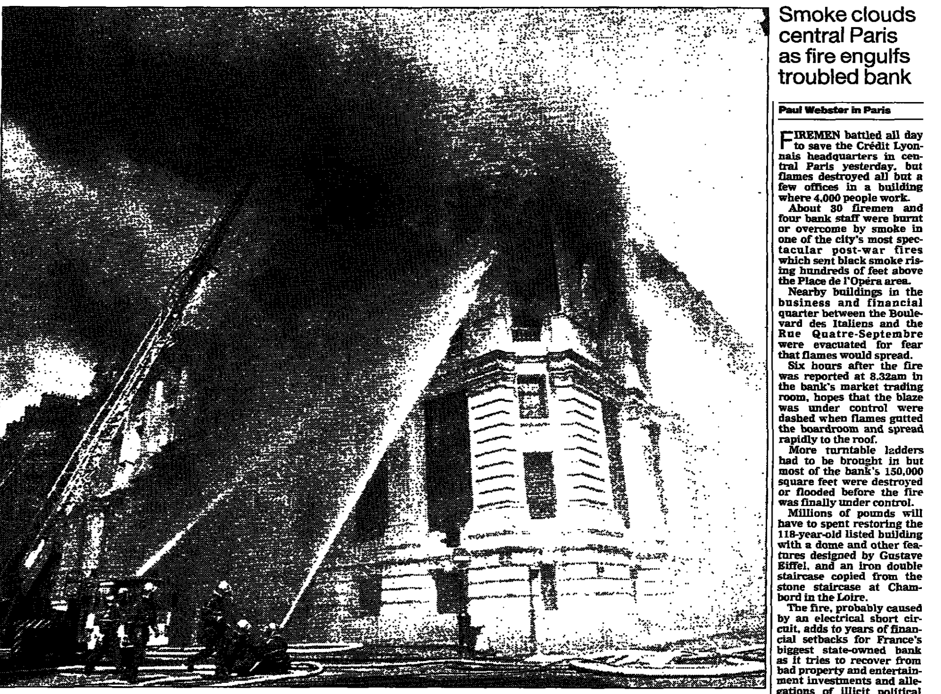
Gutted... Firemen spray water over the headquarters of the Crédit Lyonnais bank near the Place de l'Opera in Paris yesterday PHOTOGRAPH: FRANCIS MOR
